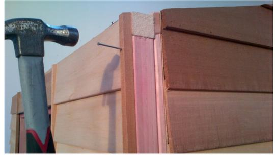
Step 12: Silicone and nail corner clashings on all corners as shown using 5 x beading nails per clashing. Note short clashings at the front, long clashings at the rear.
