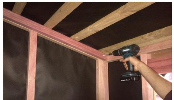
Step 15: Using 2 x 75mm framing nails, nail centre roof purlin to front and back top plate stiffeners. Pre-drill if necessary.
