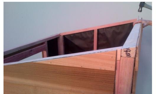
Step 10: Using 30mm Galv Clouts nail top cedar boards to stiffeners (2-3 per board). Pre-drill holes to stop boards from splitting.
