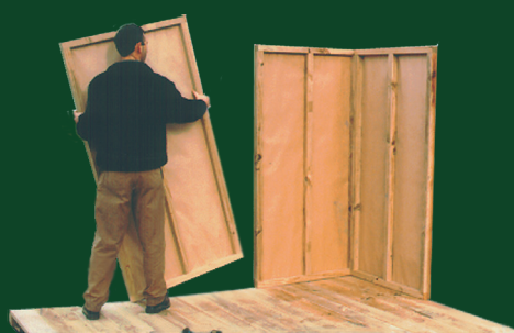
Shed assembly, erecting wall panels.
