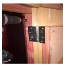
Step 22: Screw padbolt as shown, to the edge of the trailing door, (Left hand door) ensuring padbolt will protrude at least 10mm into Bottom plate in locked position.
