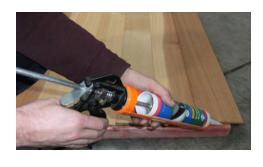
Step 7: Silicone and nail remaining beads on each panel. Screw panels together using 3 Tek screws per join and 4 on the longer joins on gable end panels.
