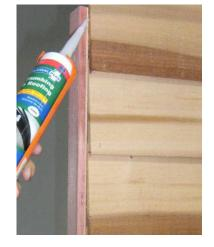
Note: On standard panels only, top of bead is bevelled to allow for slope of roof.
