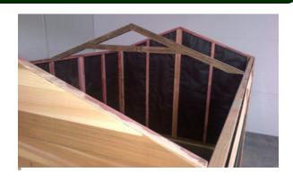
Step 14: Position 12 purlins on roof. Top purlins should be together and bottom purlins should be against top plate. Using 75mm framing nails, predrill then nail purlins into top of gable end panels and truss (2 nails per join).
